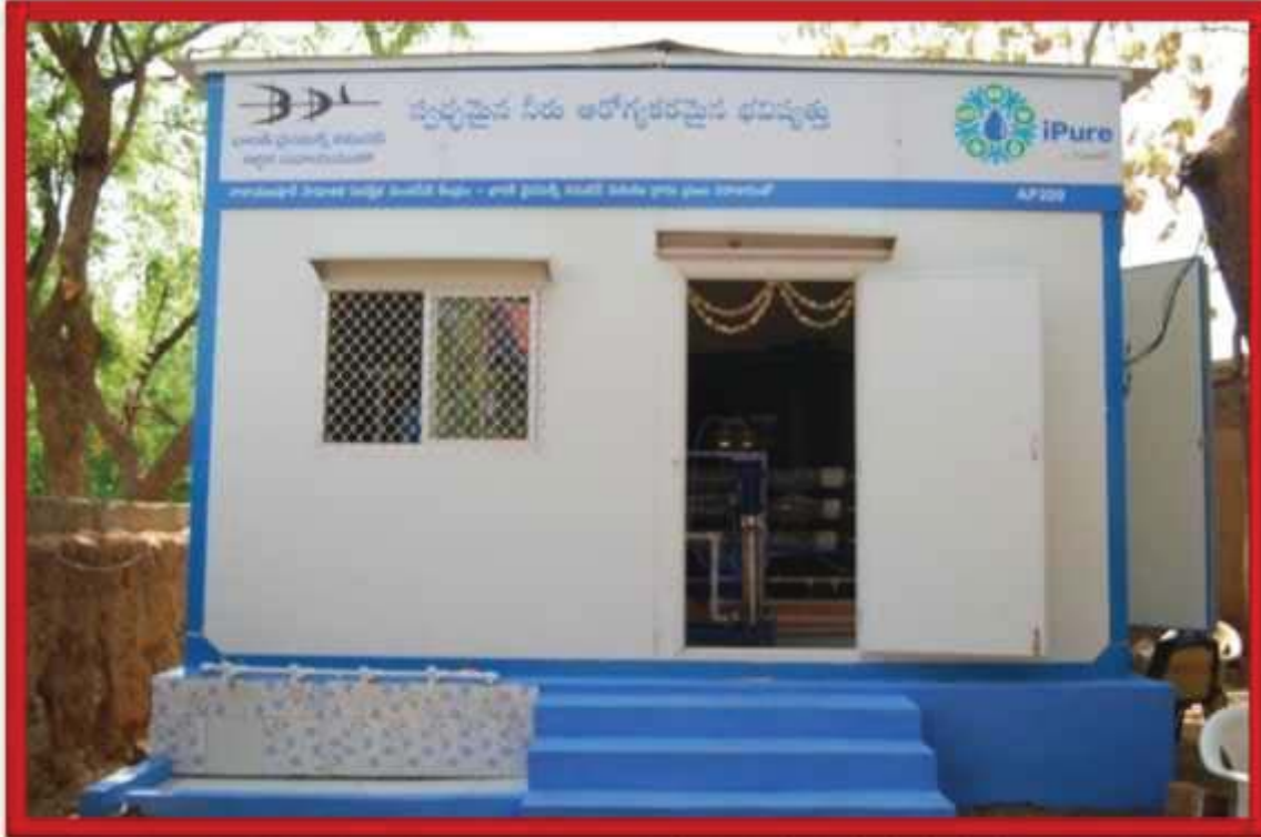
R O Water Plant at Narayanpur
