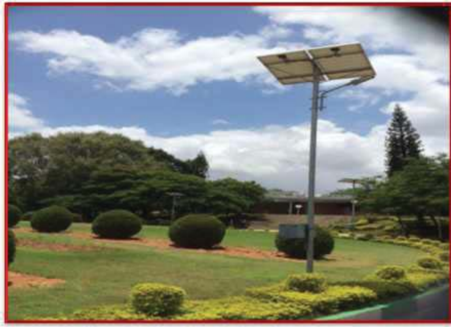
Solar street lights
