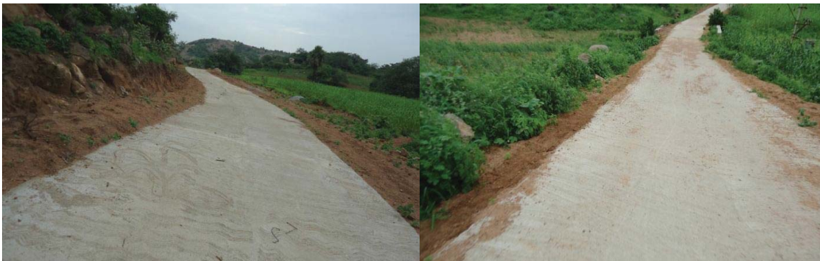
The road constructed by BDL
