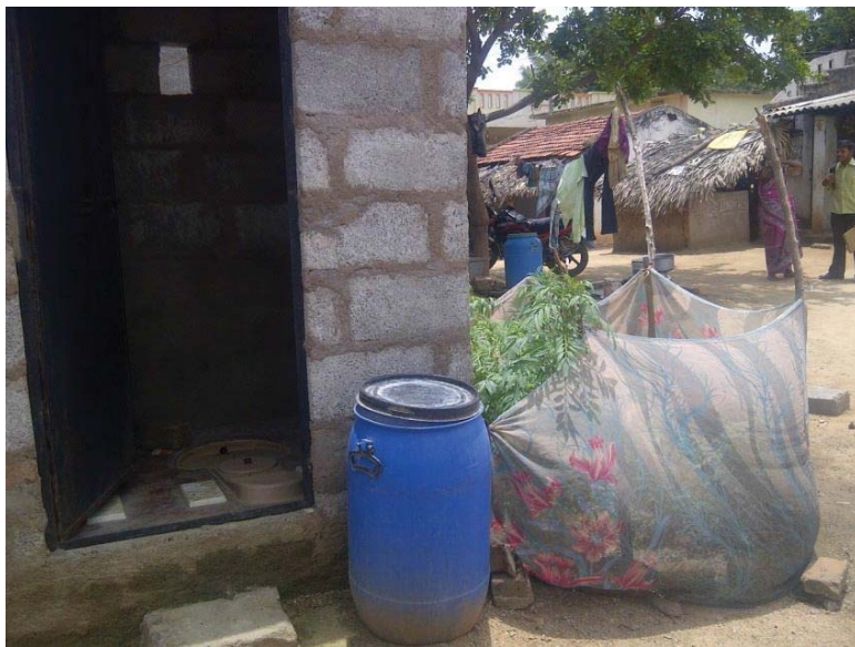
Eco sanitation toilet built by BDL
