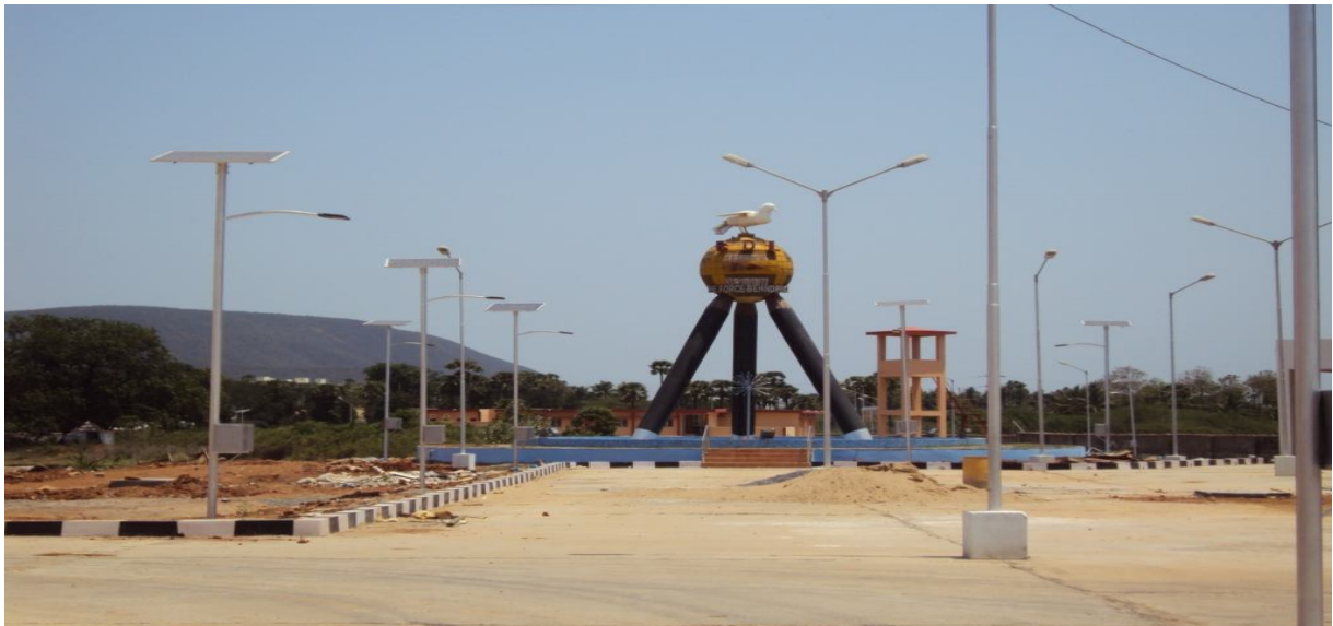
Solar street lights near Pylon and on 12mtrs Road at M/s. BDL, Vizag unit
