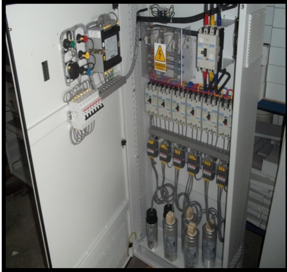
Automatic Power factor Control panel (Typical)
